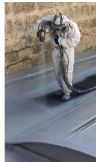
Roofs, Balconies and Terraces Dachy, balkony i tarasy
